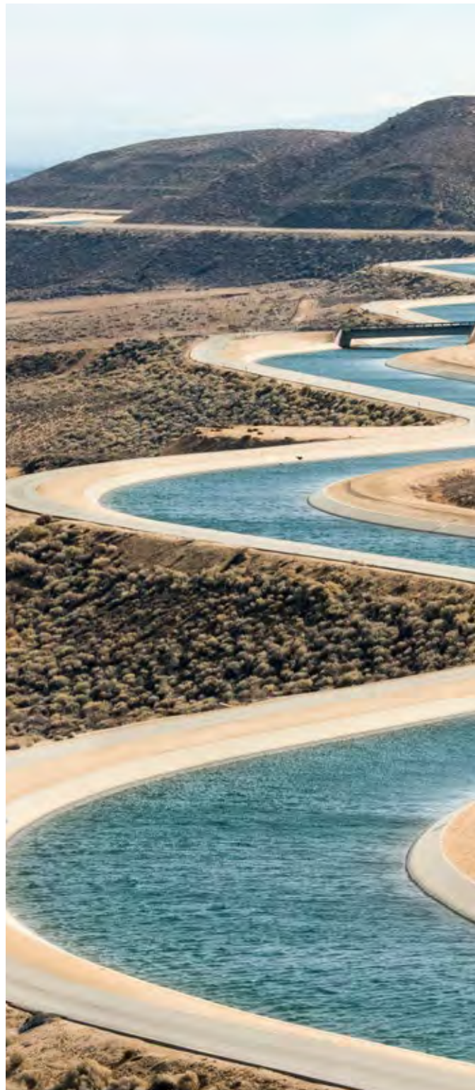
The State Water Project canal, a major conduit for imported water for the Basin.
